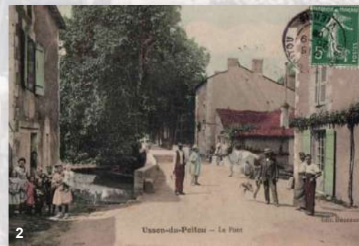
2. The bridge and the shower-baths, lean-to covered with red tiles Old postcard - Private collection
