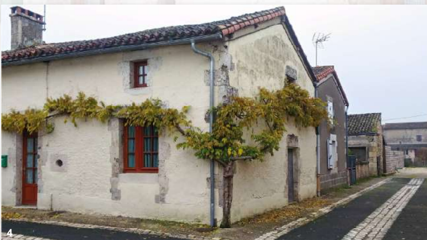
4. A restored house. The limestone frames of the openings, the angle chaining, the boulite have been preserved. The flowers add to the charm of this house Photo Ecomusée, Monique Roulet-Caire
